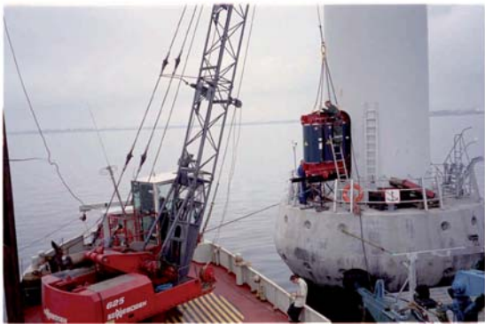
Figure 10: Transformer passing the door in the tower.
