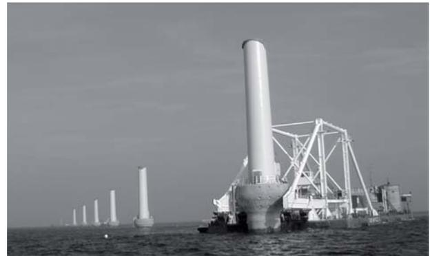
Figure 7: The floating crane with a foundation and the lower part of the tower at the site just before installation.
