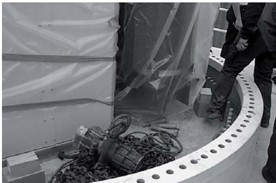
**Figure 8:** The switchgear and transformer on top of the concrete foundation ready for placement of the tower.
