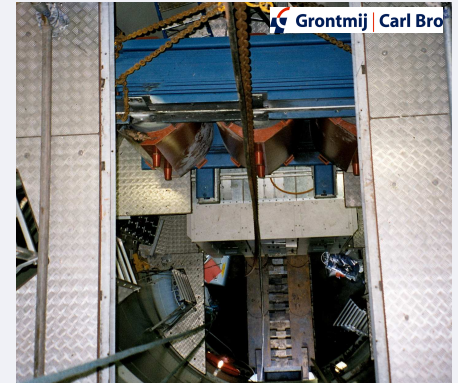
Fig. 3 Looking down at the transformer after dismantle of 3. floors inside the tower.
